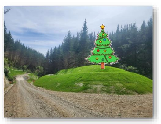
Anaura Bridge 2. The second bridge along Anaura Rd to replace a C.G. damaged culvert has been a resounding success, the bridge will also accommodate transporters as it is rated to 95T. In the periphery of the bridge, the hydroseeded slopes are noticeably green highlighting the success of the hydroseeding operation. The hydroseeding provides a fast growing vegetation cover to the slopes mitigating risk of erosion.
